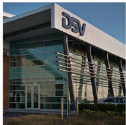
4. DSV 7 Landing Drive
